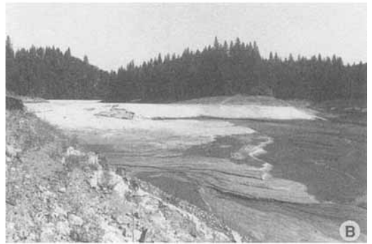
Figure 12. Dam on Greenhorn Creek, photographed around 1939. The dam is now completely buried by mining sediment indicating a substantial influx of sediment since that time. (Photograph by U.S. Army Corps of Engineers.)
