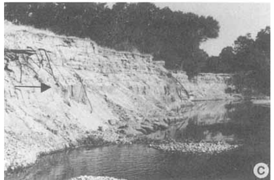
Figure 13. Views of upper Bear River showing evidence of sediment transport. (A) Terrace scarp along Greenhorn Creek showing typical erosion of tailings next to bedrock-floored channel bed. Lack of sediment accumulation indicates sediment transport out of the reach. (B) Large delta forming in Rollins Reservoir at the mouth of Greenhorn Creek. Lithological compositions indicate that the delta is comprised primarily of mining sediment. (C) Eroding bank at bend in the lower Bear River (1985). Severe erosion was observed at this site between 1983 and 1986. Mining sediment contributes a substantial portion of the sediment load. The contact between mining sediment and the underlying pre-mining soil is shown at the arrow.
