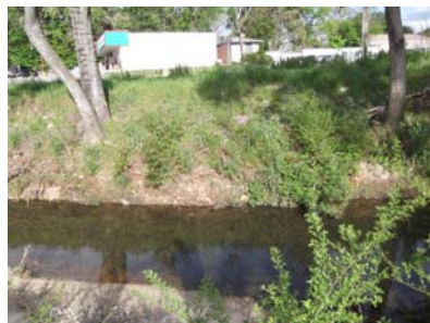
Sight 8, Bank 2: Bank slope greater than 45 degrees and 26%-50% ground cover. Is prone to erosion. B2
